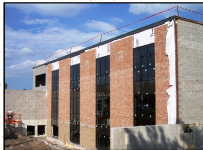
West side (Main Street) of building
